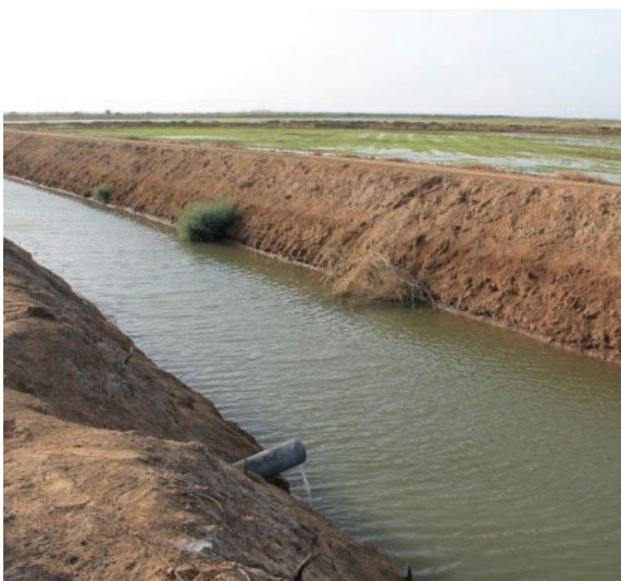
Discharge of saltwater loaded with pesticides from irrigated rice fields in the delta. Photo: Aude N. Taïbi
