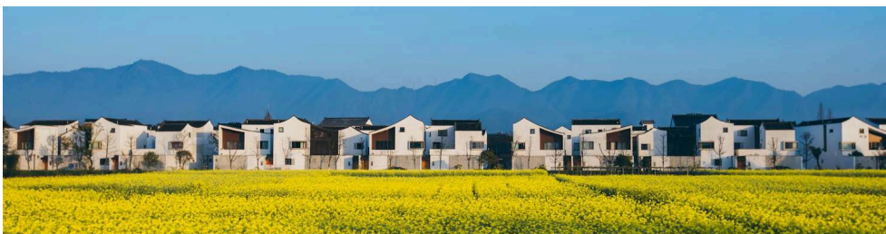
Figure 19. Façades du village Dongziguan
