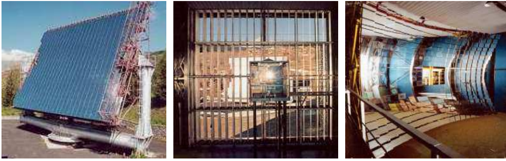
Figure 3. Main Solar Furnace (reflector, modulator, concentrator)
